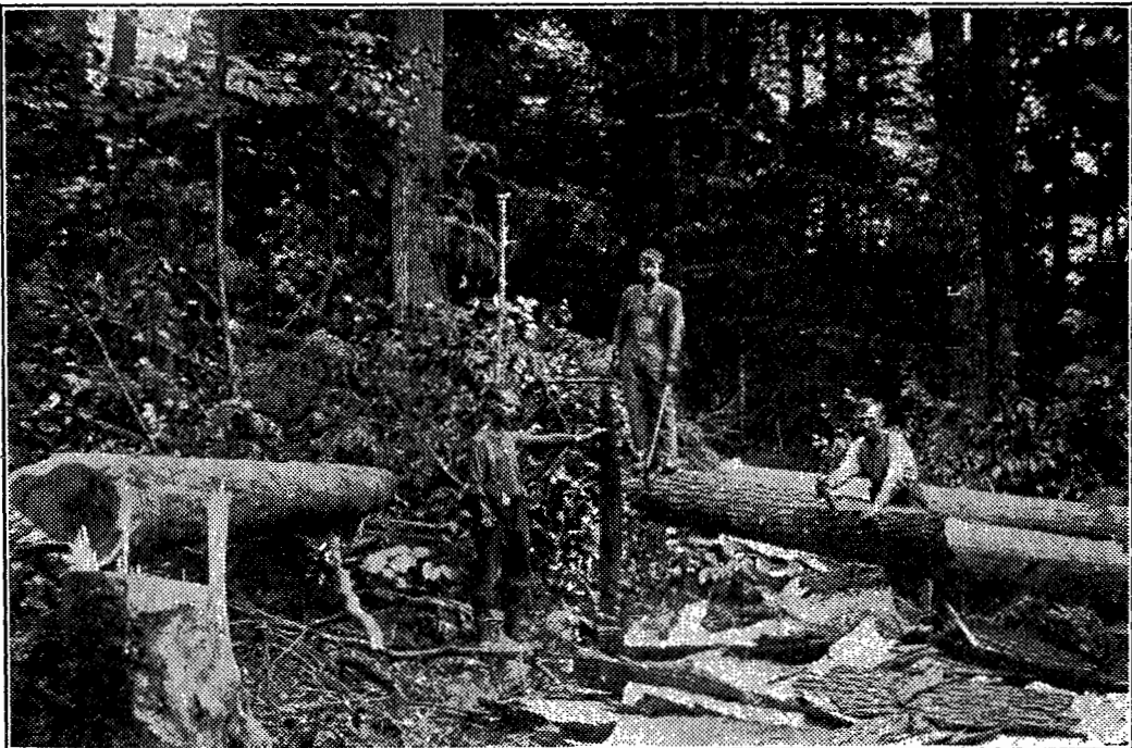
PEELING HEMLOCK BARK On Will Hartwick's job at Lyman Run
